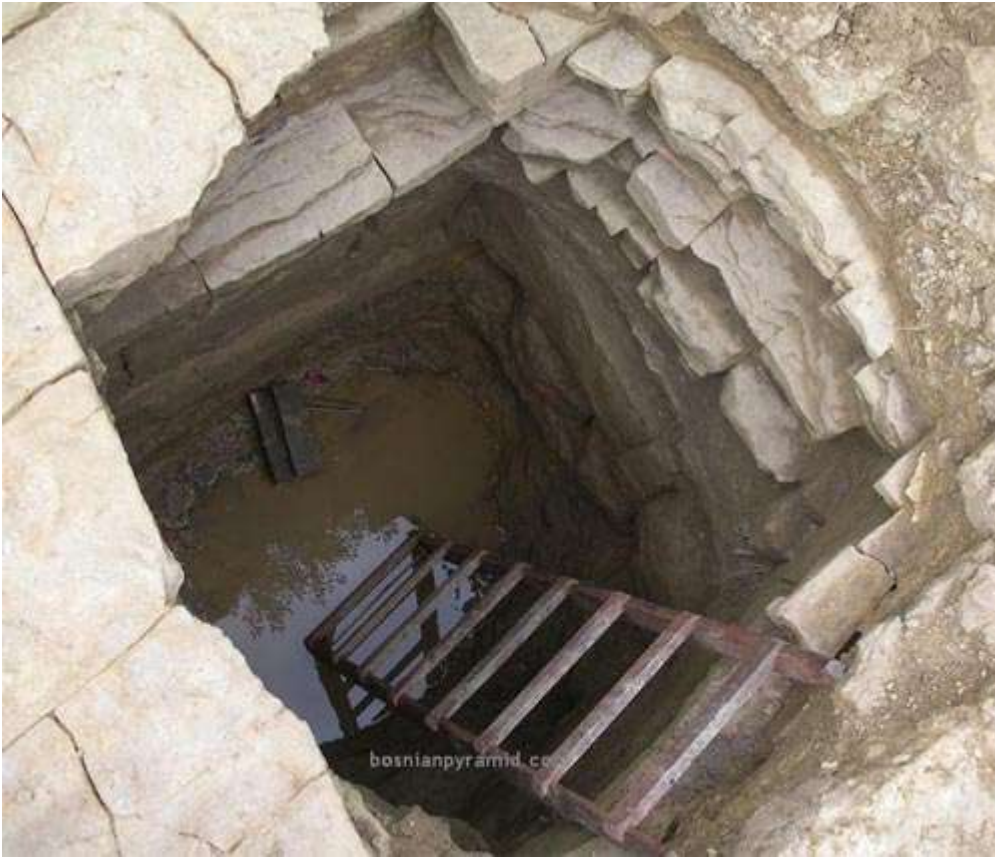
The hole has been constructed out of sandstone blocks.
